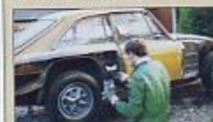
Liberal anti-corrosion protection was applied before the glassfibre rear wings were fitted.
