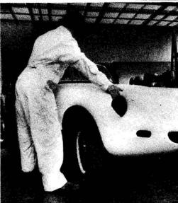
a right and a wrong way to do it. The right way is to leave a margin of 2in of metal up the trailing edge of the doors so the new glassfibre can be bonded successfully and you retain strength where strength counts. You leave the big, broad sill alone of course — unless you expect to fit really big rubber then you flatten the wheel arch edges back a little by gentle hammering and shave the glassfibre to match. But more of that later.
